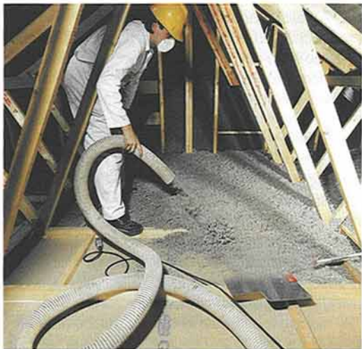
BELOW Warmcel insulation is manufactured from recycled newspaper and is claimed to be a better than carbon zero insulation
